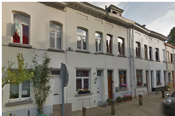
Figure 6: Workers row house – rue Jean Deraeck - 1150 Brussels
