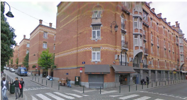
Figure 6: Social multifamily dwellings «cité Hellemans», Marolles district, Brussels (1912) (source: Google Maps)
