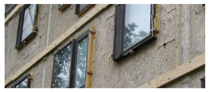
Figure 73. Old windows kept in place for a period of time, after the removal of the external layers of the existing walls (Riihimäki, FIN)
