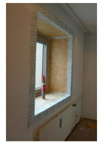
Figure 120. Tape used for airtightness around windows, <u>Berlin</u> (DE)
