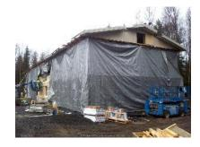
Figure 144. Protection of installed modules before the implementation of the cladding (<u>Oulu, FIN</u>)
