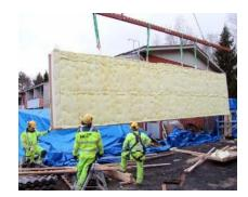
Figure 59. Example of a full-span compression layer for closed TES installed on-site in Oulu (FIN)
