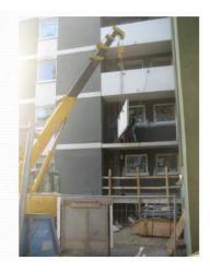
Figure 139. Part of old balconies cut down in Augsburg, DE
