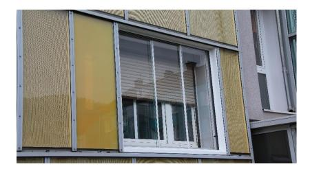
Figure 71. Conservation of the existing windows and integration of a single-glazed window into the AIMES modules
