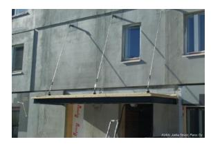
Figure 154. Additional architectural elements fixed on modules (<u>Riihimäki, FIN</u>)
