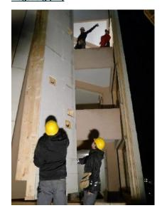
Figure 48. How the particular shape of the building (complex balconies) played a role in the choice of vertical modules orientation (Illustration: <u>Berlin</u>)
