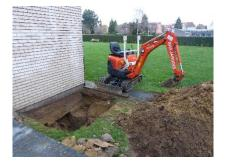
Figure 41. Excavation to characterise the foundation system
