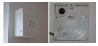
Figure 82. Decentralised ventilation unit installed on indoor walls surface (left) and without its cover (right). This technology was used In <u>Graz-1 & 2 (AT)</u>
