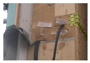
Figure 103. Rebate joint with a rubber lip for airtightness (London, UK)
