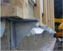
Figure 107. Mounting layout used in Graz-1 (AT) (top) Vertical attachment substructure; (bottom) large brackets to collect loads at base.
