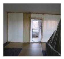
Figure 136. Dust screen installed to protect the indoor spaces during onsite interventions (Berlin)
