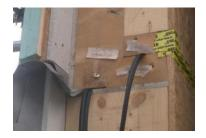
Figure 122. Rubber lips and tape to limit wind penetration between modules (London, UK)
