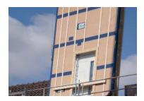
Figure 121. Tape used for wind protection to avoid the penetration of exterior air between the exterior panels of the AIMES element, Roosendaal (NL)
