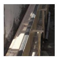
Figure 125. An example of moisture-safe design: moisture barrier between the footing and the base sill of the wall
