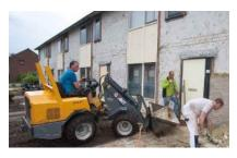
Figure 138. Partial removal of the existing cavity walls (<u>Roosendaal, NL</u>)
