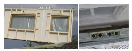
Figure 86. 'TES-connected' system with ventilation ducts incorporated in the new envelope in <u>Zurich, CH</u>. (left) Ducts integrated in a special fire-proof casing inside AIMES modules; (right) view of the top of one AIMES element showing the ventilation ducts
