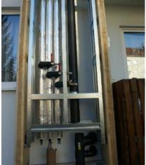
Figure 78. Installation duct (left) Section of an installation duct: (A) insulation; (B) duct work; (C) panels, fire protection. Source: [1]; (right) Example in Kapfenberg (AT)
