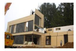
Figure 51. Use of AIMES modules for balcony incorporation in <u>Augsburg, DE</u> (left) or to create a new storey in <u>Pettenbach, AT</u> (right)
