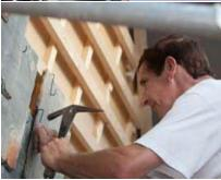
Figure 153. On-site fixation of external layer (top) Trespa panel in Berlin
