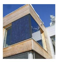
Figure 90. PV panels integrated in AIMES modules (Pettenbach, AT)
