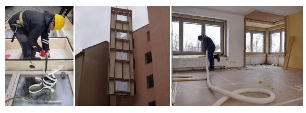
Figure 64. Mineral wool flakes blown into the timber elements after assembly in Berlin (DE) (left) Installation of 'compriband' on the back of the open TES (middle) Lifting of a module before installation (right) Injection of the insulation material from the inside
