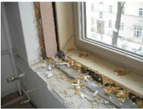
Figure 152. Insulation injection for Open TES modules (top) <u>Pettenbach, AT</u> (bottom) <u>Berlin, DE</u>
