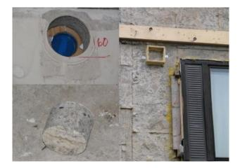
Figure 143. Holes drilled in the existing walls to connect the ventilation ducts (Riihimäki, FIN)
