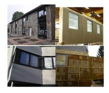
Figure 65. Various solutions for the external layer (top-left) Natural slates in Roosendaal, NL; (top-right) plaster in Riihimäki; (bottom-left) HPL panels in Berlin; (bottom-right) 'Solar façade'
