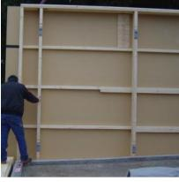
Figure 113. Hook in system used in Pettenbach
