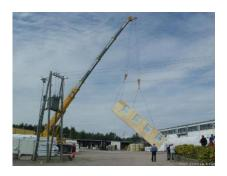
Figure 149. Tilting of modules in Riihimäki (FIN)
