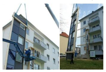
Figure 129. Prototype module implemented in Kapfenberg (AT) before the actual execution
