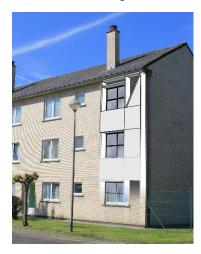
Figure 1. Principle of prefabricated envelope modules projected on an existing building
