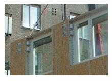
Figure 80. Decentralised ventilation ducts pre-fitted in the modules.
