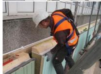
Figure 150. Fixation of the module to the attachment substructure: <u>Augsburg</u> (<u>DE</u>) and <u>London (UK)</u> cases show a similar fixation method
