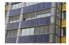
Figure 88. PV panels integrated in AIMES modules (Graz-2, AT)
