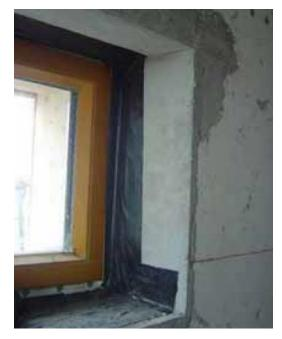
Figure 156. Installation of airtightness tape in Pettenbach (AT)
