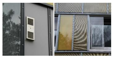
Figure 84. Apparent air inlet and outlet of decentralised ventilation units (left) or hidden behind glazing (right).
