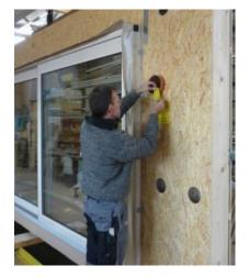
Figure 130. Application of an airtightness tape around integrated ducts (<u>Augsburg</u>, <u>DE</u>)
