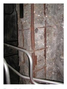
Figure 40. Exposed concrete reinforcement. Source: [13]
