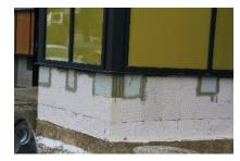
Figure 108. Bottom XPS insulation in front of the large brackets used to collect loads at building base (<u>Graz-2</u>,
