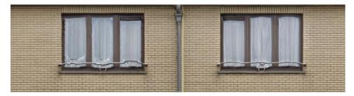
Figure 36. Deformations on the cloud point produced by the SFM method, due to reflective materials (Brussels case study)
